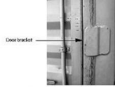
Using both hands, secure the device on the left door until it is flush.
